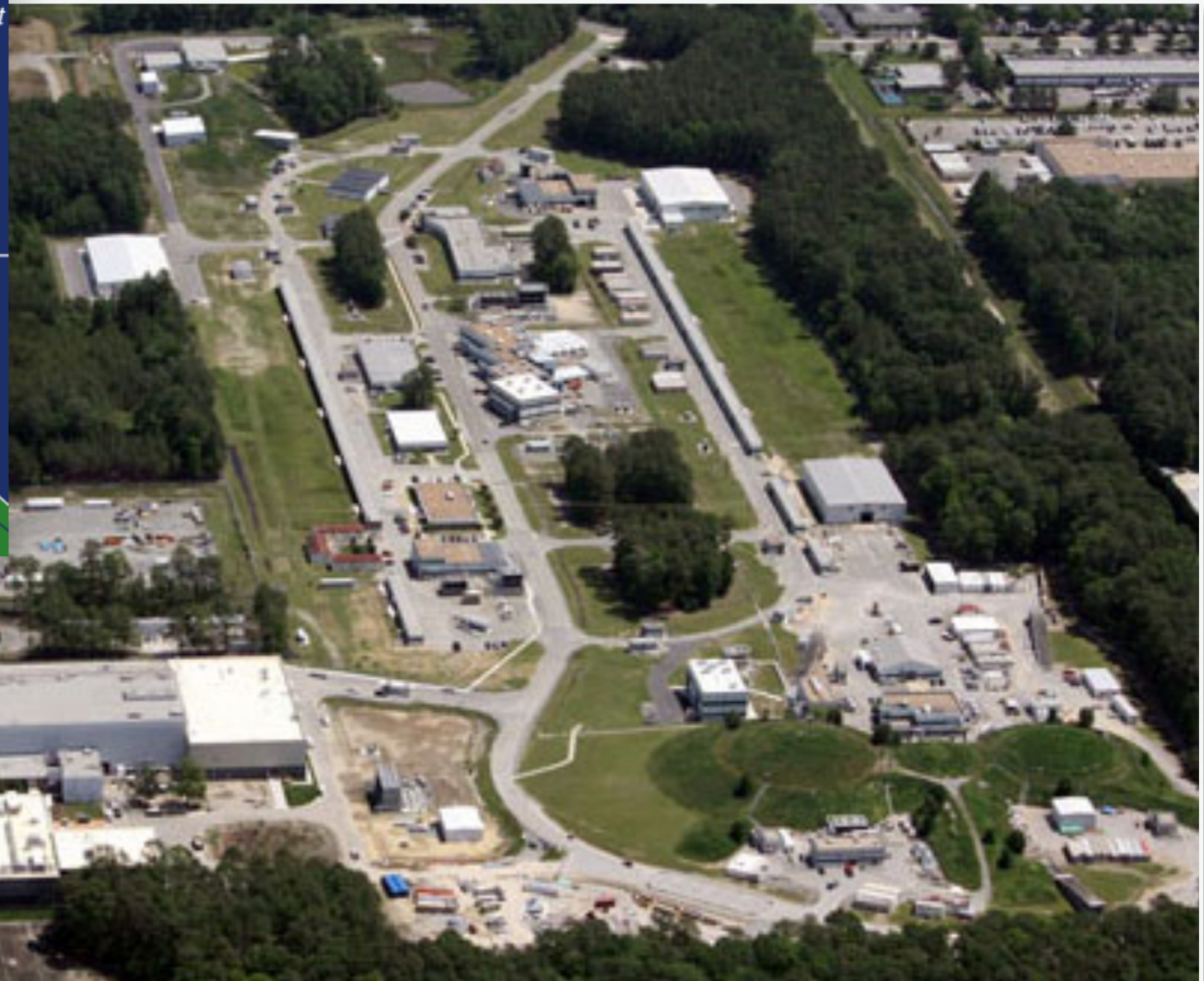
Continuous Electron Beam Accelerator Facility (CEBAF) at Thomas Jefferson National Accelerator Facility
