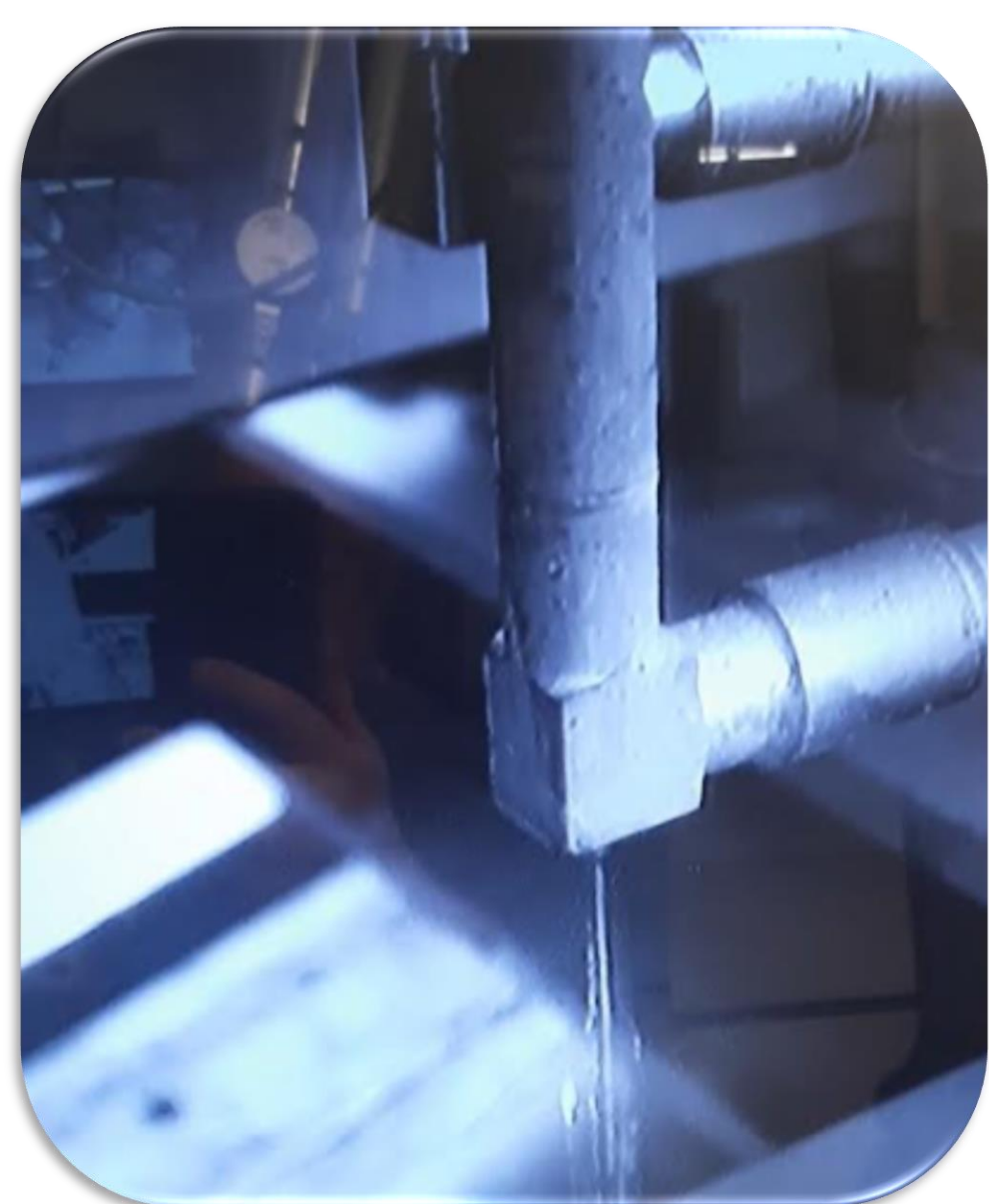
(a) Visual leak spotted on the vertical pipework below the pre-moderator (left). (b) Remote handling visual inspection showing a small amount of corrosion around electron beam welded pip weld (right).
