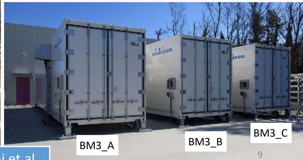
Capacitor Banks for BM3
