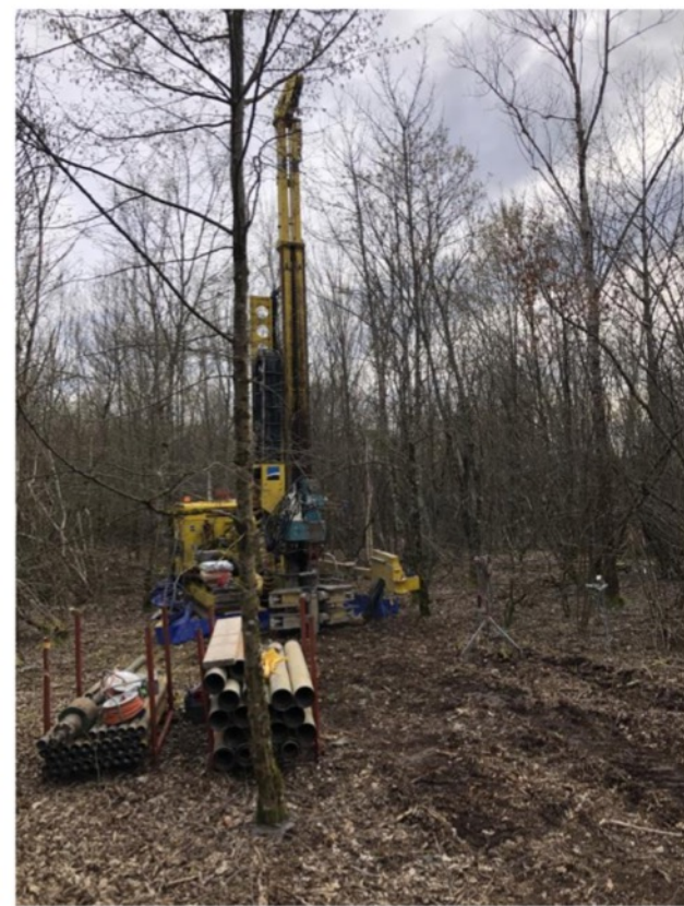
➤ Drilling machine in place
